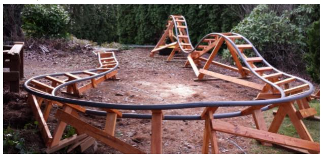
Track width and cart length are important decisions. Track width is based on intended rider weight and height. If the rider is larger and taller, a wider track width is needed, to accommodate a longer cart, and to better handle a higher center of mass. Tracks for lighter, shorter riders can have narrower track width (gauge) so the cart can be shorter, which means the track turn radii can be smaller, and the track fits in a smaller space.
